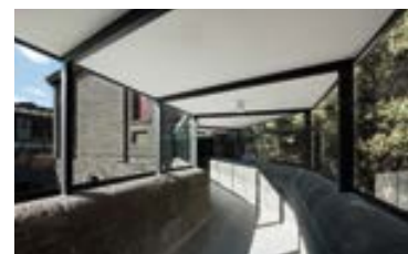
The refurbished Old Melbourne Gaol Gatehouse.
