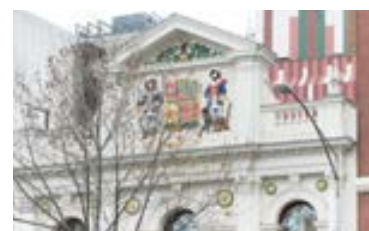
Refurbishment of the 1888 home of the Ancient Order of Foresters returned its facade to original condition through rich detailing and decoration.
