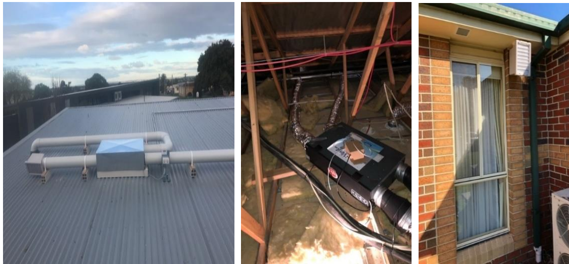
Figure 7 (1) Roof installation, (2) Ceiling installation, (3) External filter box installation (Source: Eco Pacific)
