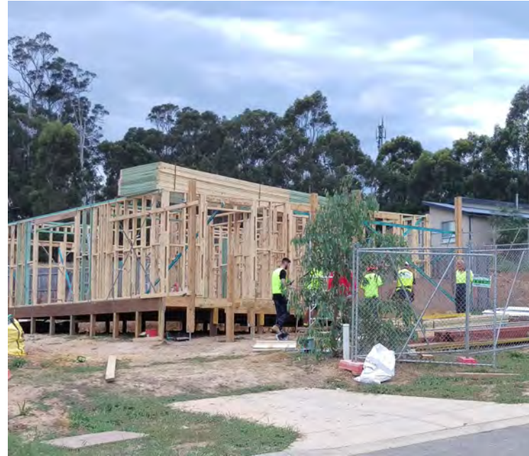
Construction of frames for Habitat for Humanity, Yea
