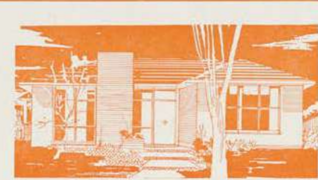
V337 This house is a contemporary version of V324. Its shallow roof would be ideal for one of the new patented steel roofs which are fixed by the manufacturer and therefore very suitable to be used by owner-builders. This plan contains the most popular bathroom arrangement. The shower recess is separate from the bath and the w.c. is off but has an additional external doorway. The bath is set in a bench top. Just over 12 squares it will fit on 50' block or across 55'. With the alternative placing a different position for the front entrance should be considered. Current estimate £3400.
