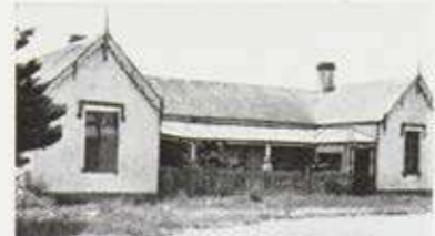
C.1850. INFANCY: SINGLE-ROOM-WIDTH WINGS FORM AN OPEN COURTYARD; A NARROW INTERNAL VERANDAH GIVES ACCESS TO THE ROOMS; JUST SOUTH OF GEELONG, IN WHITE STUCCO ON HANDMADE BRICKS.
