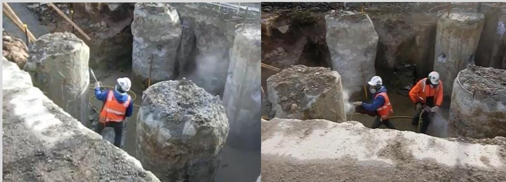
Figure 3.1: Using a hand-held pneumatic breaker to break down concrete pile heads
