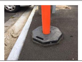
Two bases fitted to prevent bollard blowing over in the wind
