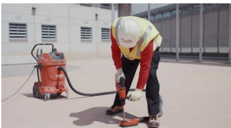
Concrete drilling using Hepa filtered vacuum extraction.
