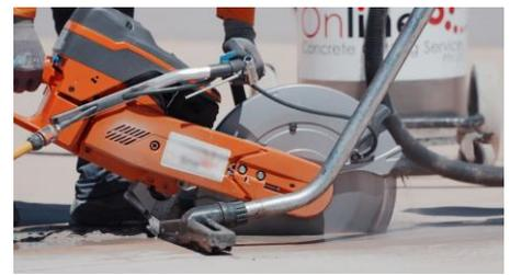
Concrete cutting and cleanup using on-tool water suppression, dust extraction, and vacuuming.
