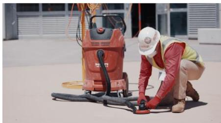
Concrete grinding using Hepa filtered vacuum extraction.
