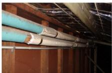
Asbestos pipe insulation may be concealed under layer materials and wrappings.
