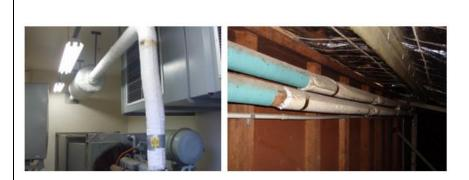
Asbestos pipe insulation may be concealed under layer materials and wrappings.
