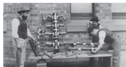
A plumbing instructor preparing samples for students.
