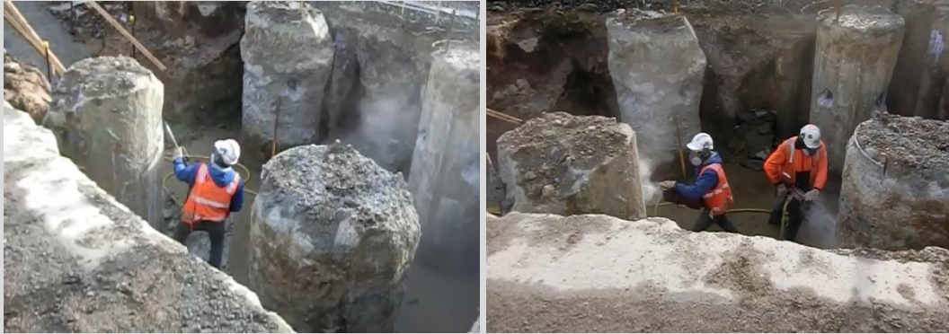
Figure 5: Using a hand-held pneumatic breaker to break down concrete pile heads
