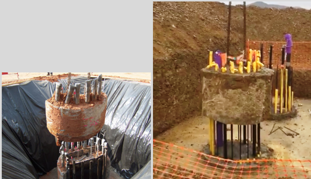
Figure 6: The Recepieux pile breaking method
