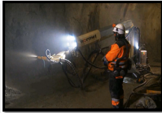
Mechanised shotcreting
