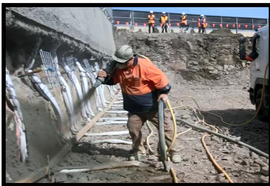
Manual hand-held shotcreting
