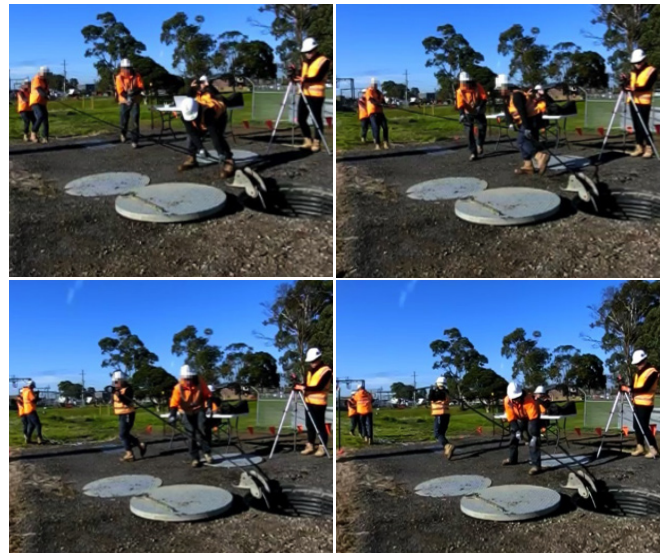
FIGURE 4: Cable pulling involves bending of the back and application of considerable force REFERENCE(S): 6.1.3, p. 146.*
