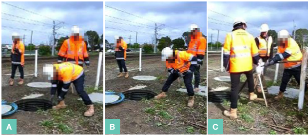
FIGURE 7: Cable-pulling without the trestle (A) and (B), compared to cable-pulling with the trestle (C).*
