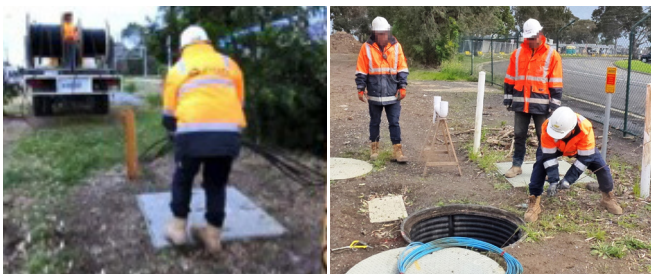
FIGURE 1 AND 2: Cable pulling preparation and set up REFERENCE(S): 6.1.1, p. 146.*
