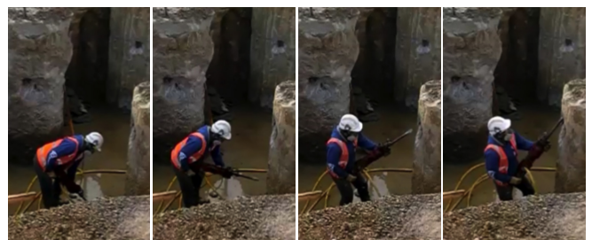
FIGURE 2: Lifting the jackhammer into position* REFERENCE(S): 7.2.2, p. 175.
