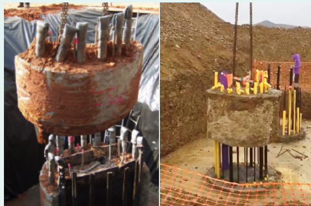
FIGURE 4: Alternative chemical pile breaking method 3
