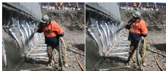
FIGURE 5: Manual shotcreting* REFERENCE(S): 5.3.2, p. 131.
