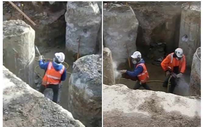
FIGURE 1: Breaking the top of concrete piles using a jackhammer* REFERENCE(S): 7.1.5, p. 173.
