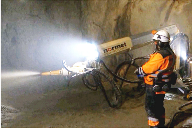
FIGURE 8: Robotic application of wet shotcrete (image courtesy of Normet Asia-Pacific Pty Ltd)
