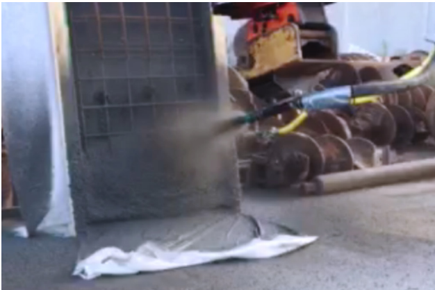
FIGURE 7: Excavator mounted shotcreting (image courtesy of Acciona Geotech Holdings)
