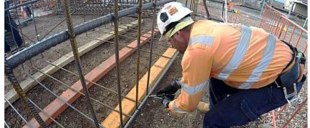
FIGURE 3: Steel-fixing at ground level*
