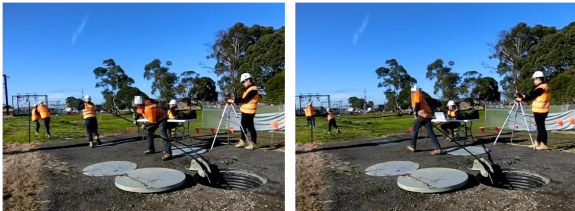
Figure 6.18: Participant 8 pulling the cable by placing it over his left shoulder and walking away from the pit, while others assist.
