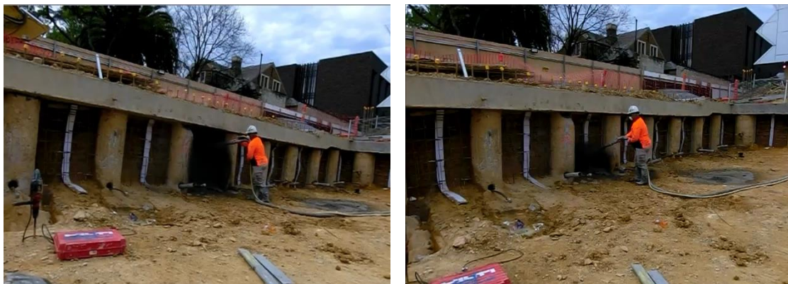
Figure 5.3: Site 5 showing the environment and participant shotcreting, and different levels.
