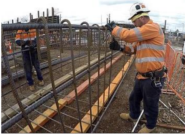
Figure 4.1: Site 1 showing steel fixing a bridge beam frame.
