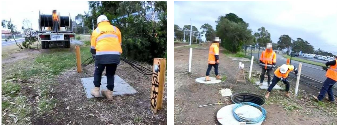
Figure 6.1: Commencing the cable pulling tasks using a standing position only.
