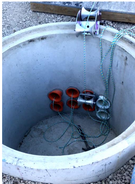
Figure 6.2: Guidance and protective devices used for ropes and cables within and on upper edge of pit.
