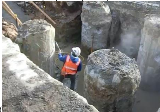
Figure 7.3: Site 3 – examples of jackhammering above ground level.
