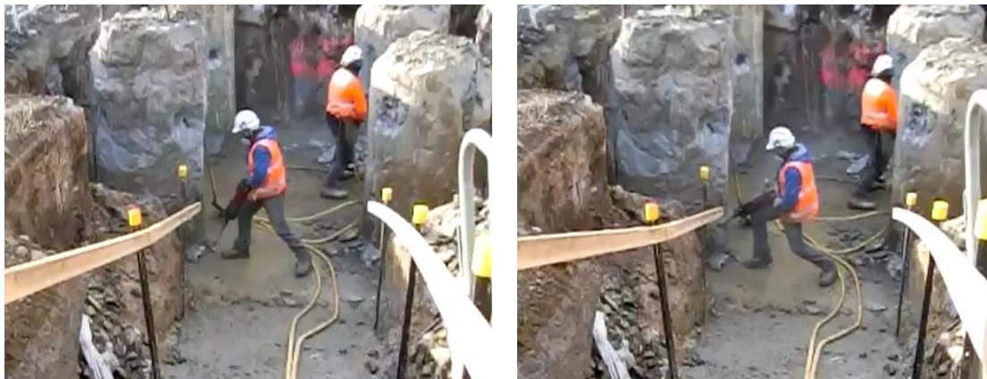
Figure 7.5: Site 3 showing handling of jackhammer tool to operate between knee and ankle height.
