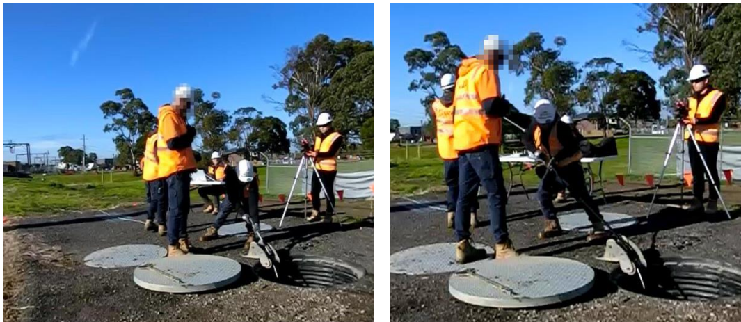
Figure 6.17: Participant 8 reaching down and then pulling upwards to pull the cable through the conduit, with observed high force exertion.
