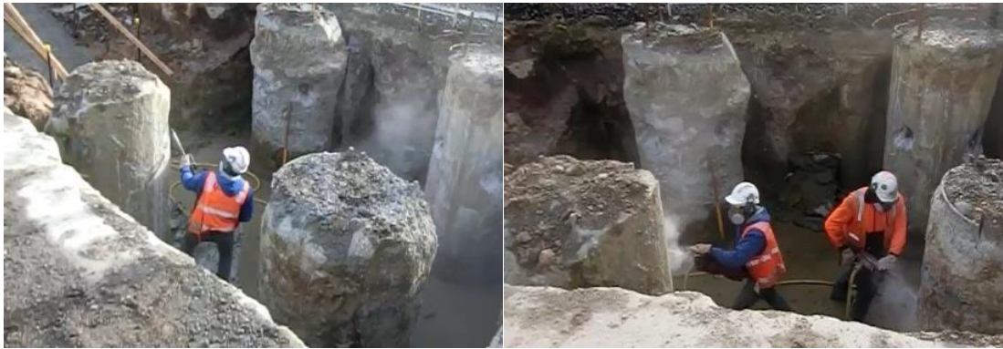
Figure 7.3: Site 3 – examples of jackhammering above ground level.
