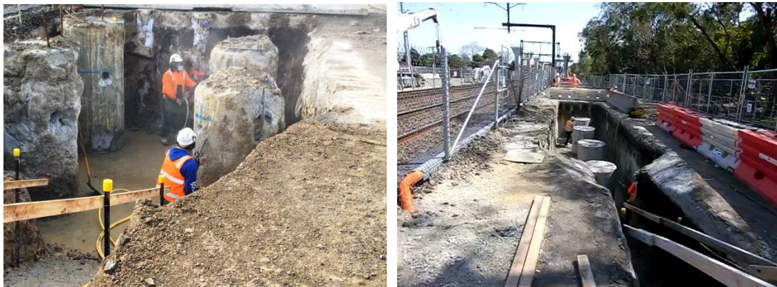
Figure 7.2: Site 3 excavations and columns on each side of the rail corridor.
