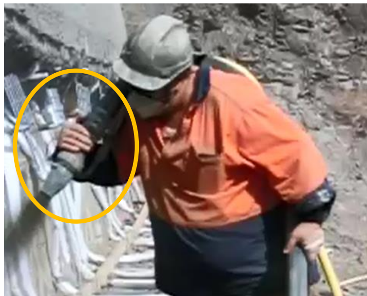
Figure 5.2: Site 7 – participant holding hose to spray concrete with no handle available or used.
