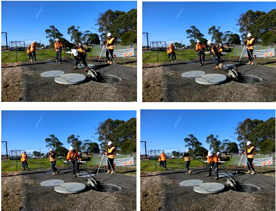
Figure 6.3: Sequence of cable pulling movements.
