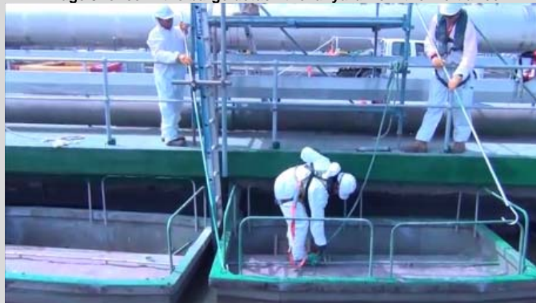
Image 10: reattach lanyard to the barge's centre safety bar
