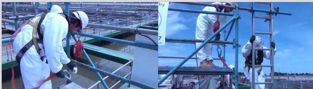
Image 7: attach the lanyard to the inertia reel
