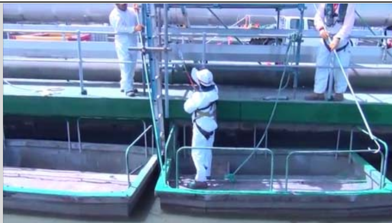
Image 9: once in the barge detach the lanyard from the inertia reel
