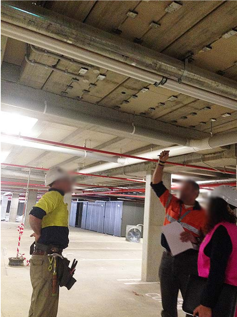
Image 19: L-R a worker, David, and Rae discussing ceiling plates and conduit
