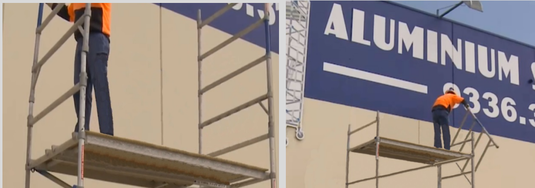
Images 1 and 2: erection of scaffolding showing the unprotected edge
