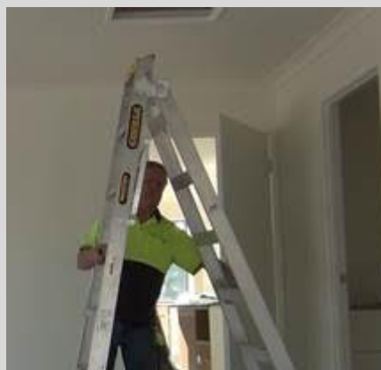
Image 13: accessing ceiling manholes using an A-frame ladder
