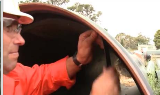
Image 17: push, compress and snap
