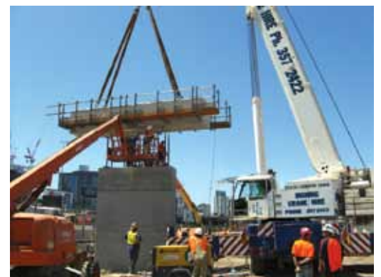
Erection of pre-cast crosshead. Photograph courtesy of: West Gate Freeway Alliance
