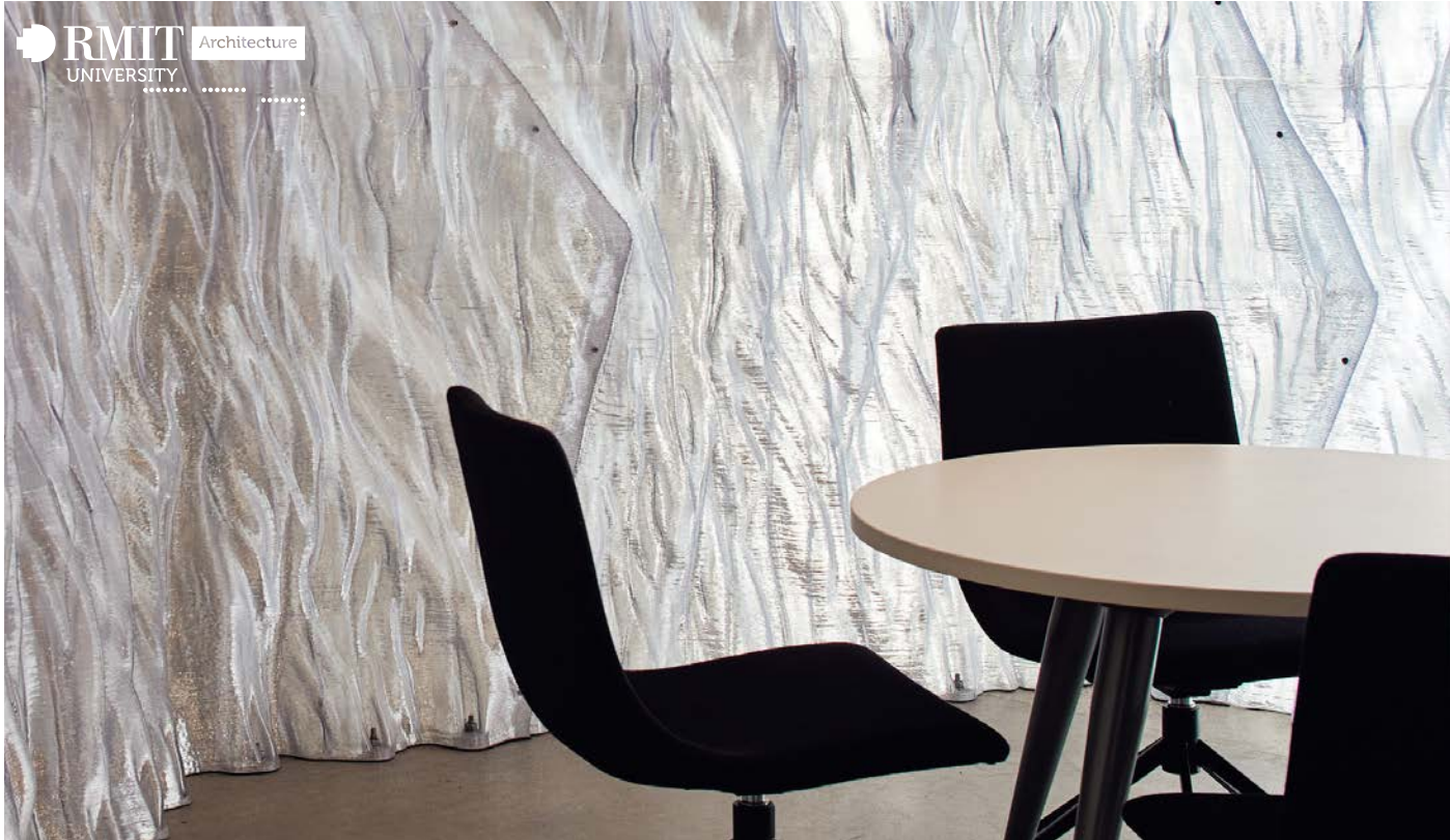
↑ 3D printed polymer walls of the SensiLab Studio. Tectonic Formation Lab 2017.
