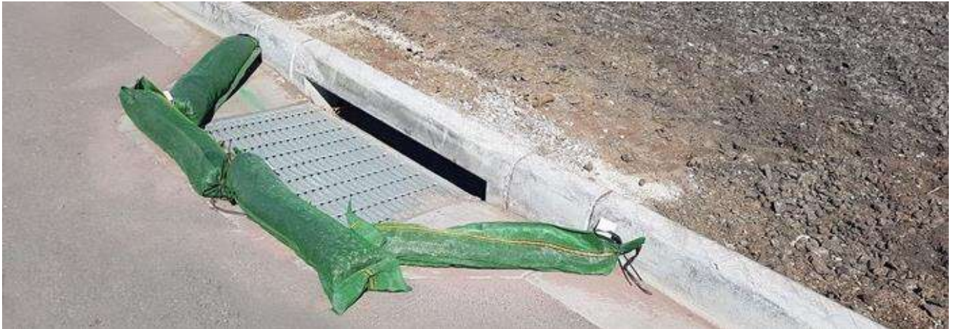
Figure 5.3. Silt sock in use to prevent sediment entering drain inlets (photo courtesy of McConnell Dowell).
