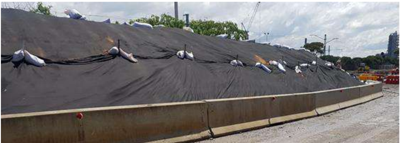
Figure 2. Covered stockpile (photo courtesy of McConnell Dowell).
