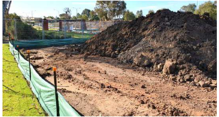
Photo courtesy of Kane Constructions.
