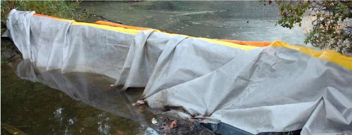
Figure 1. Engineered silt curtain installed to prevent migration of sediment for construction works within a waterway.
