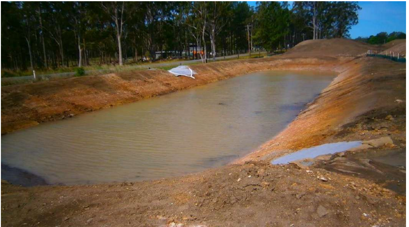
Figure 5.4. Installed sediment basin (photo courtesy of McConnell Dowell).
