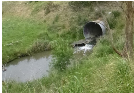
Untreated sewage can enter waterways from septic and sewer leaks, and through engineered Emergency Relief Structures during wet weather
